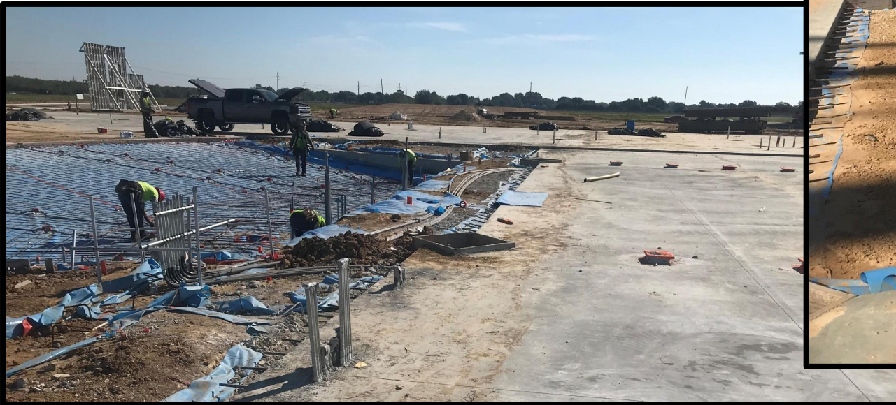
Auditorium sloped seating preparation
