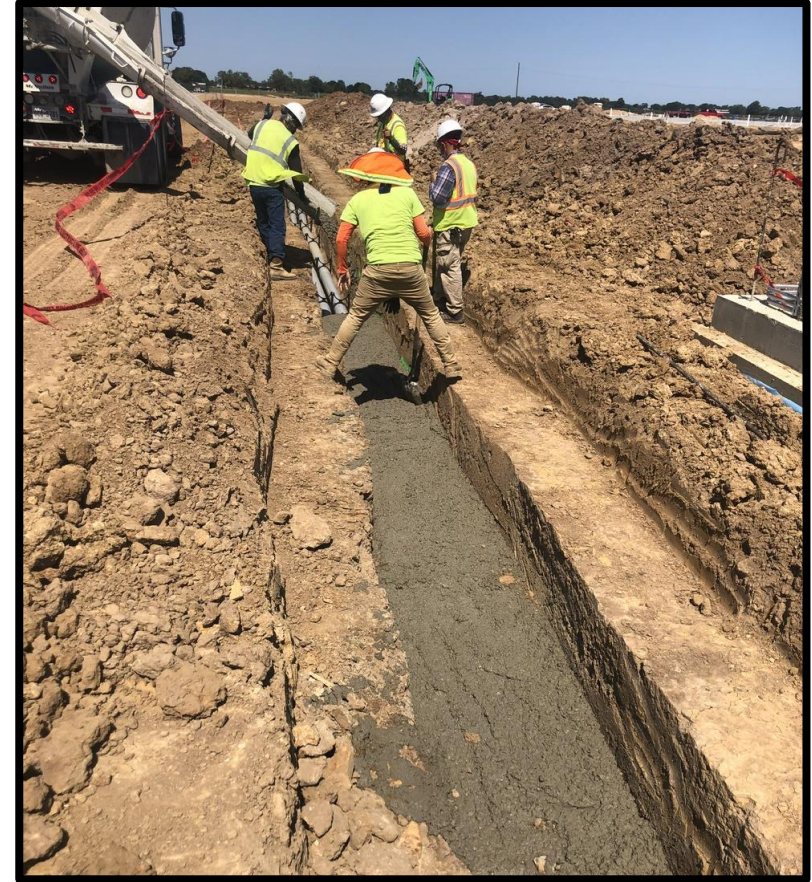
CenterPoint electrical ductbank
