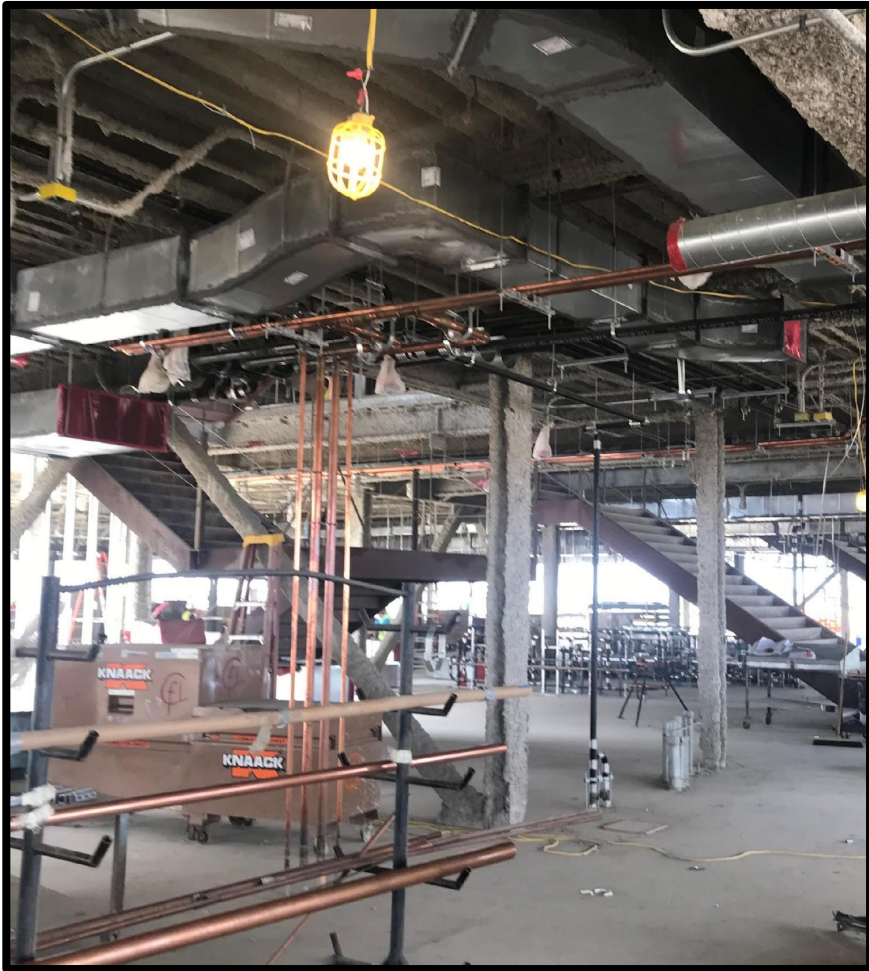
Plumbing, HVAC, and Electrical Rough-In (Fire Proofing)
