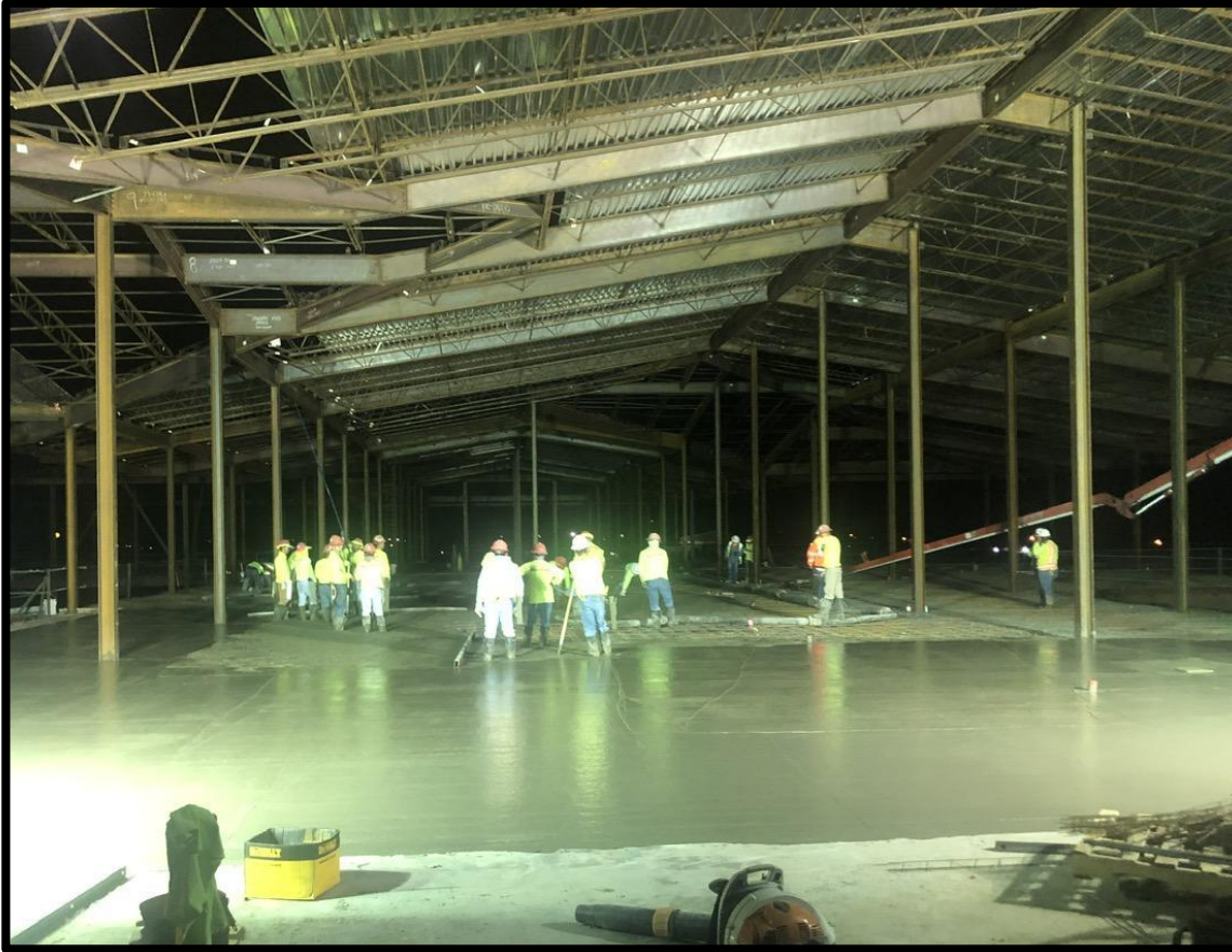
Early morning Concrete pour in Area 3 rd Floor Area E
